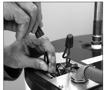
Figure 19 - Connecting the electrical wires.
