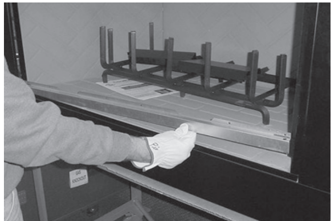
Figure 1 - Install the Door Track
