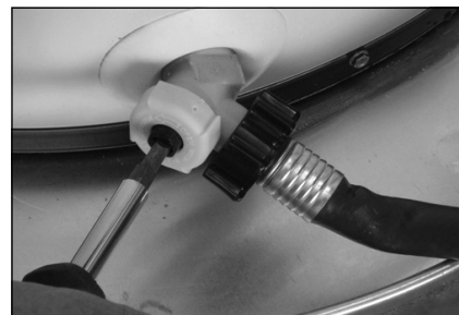
Figure 20 - Draining the old water heater.
