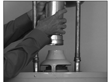
Figure 22 - Disconnect the vent pipe from the draft hood.
