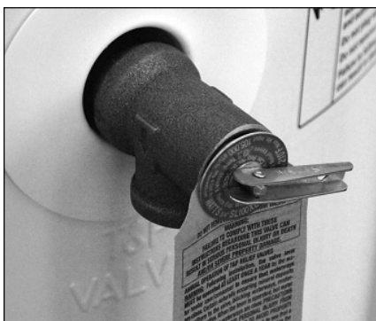
Figure 25 - Temperature and Pressure Relief Valve
