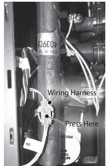
Figure 76 - Wiring harness location
