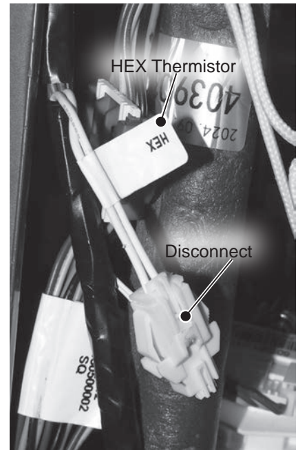
Figure 43 - Disconnecting HEX thermistor
