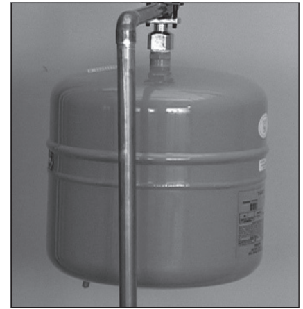
Figure 6: A Thermal Expansion Tank helps protect the home's plumbing system from pressure spikes.
