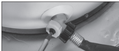
Figure 47: Draining the water heater.
