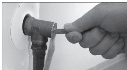
Figure 50: T&P Relief Valve.
