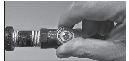
Figure 56: Gas valve in “on” position.
