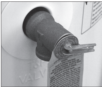
Figure 32: Temperature and Pressure Relief Valve
