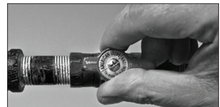
Figure 47: Gas valve in “on” position.
