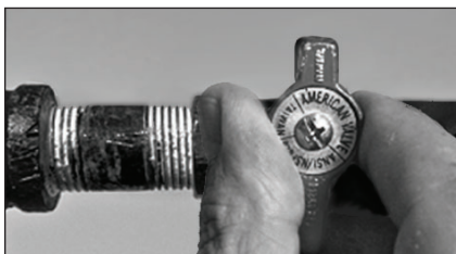
Figure 43: Gas valve in “off” position.
