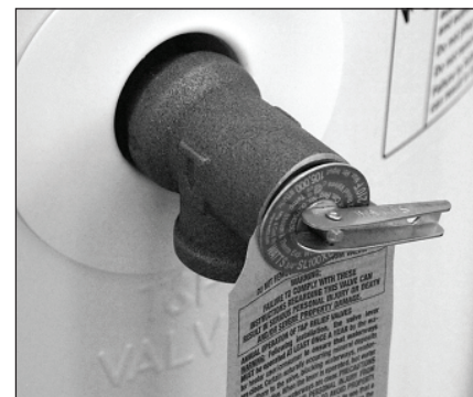
Figure 18: Temperature and Pressure Relief Valve
