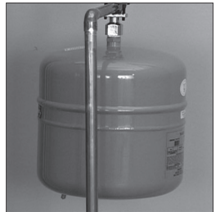
Figure 22: The Thermal Expansion Tank should be pressurized with air, using a hand pump, to match the home's incoming water pressure.
