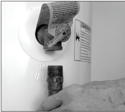
Figure 13: Removing the T&P Relief Valve discharge pipe.
