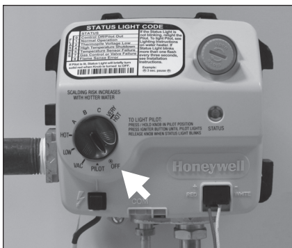
Figure 42: Gas control/valve.
