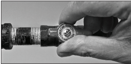
Figure 29: Gas valve in "on" position
