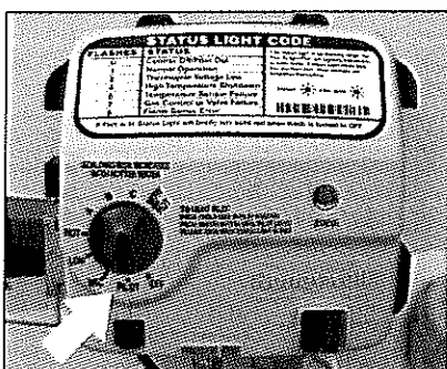
Figure 33 - Gas control/valve.
