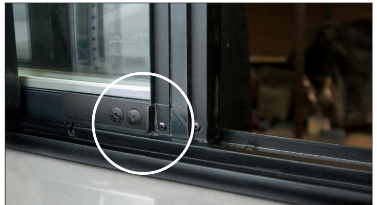
Fig. 2. Door latch is in the closed position (disengaged from notch).
