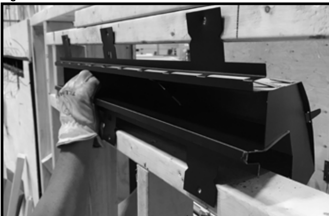
Figure 5.18 Position Plenum
