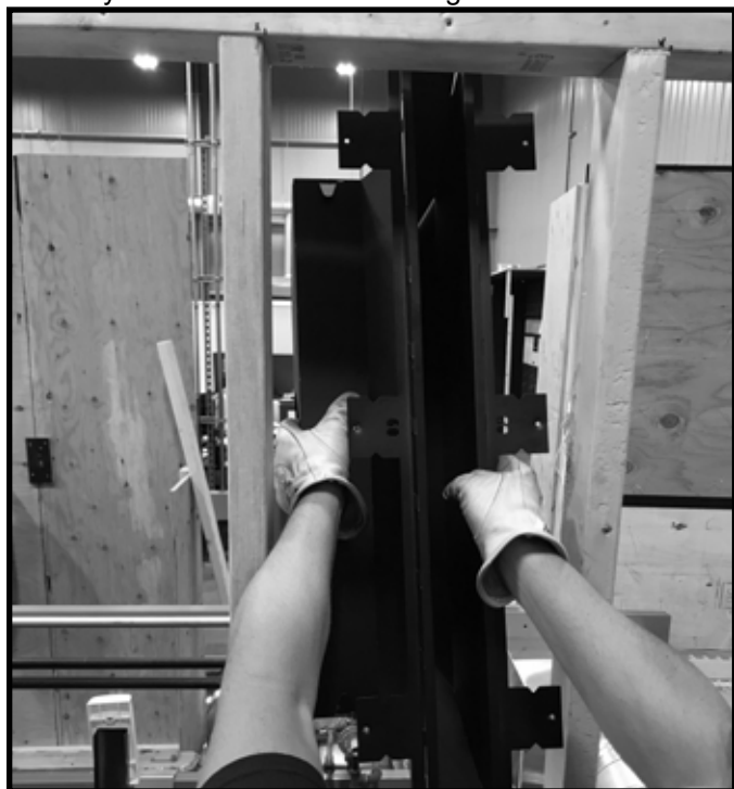
Figure 5.15 Turn Plenum Vertically to Clear Framing Studs
