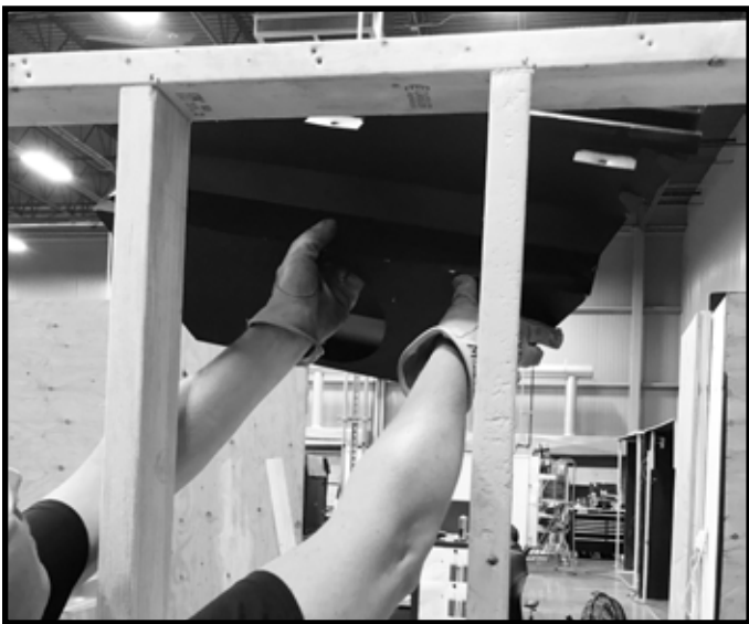
Figure 5.16 Rotate Plenum to Horizontal Orientation
