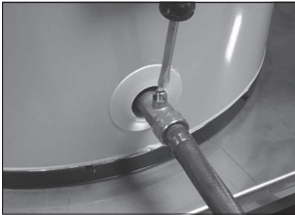
Figure 10 - Draining the old water heater.
