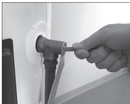
Figure 40 - T&P Relief Valve
