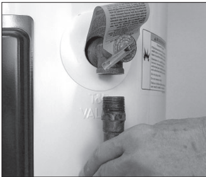
Figure 11 - Removing the T&P Relief Valve discharge pipe.
