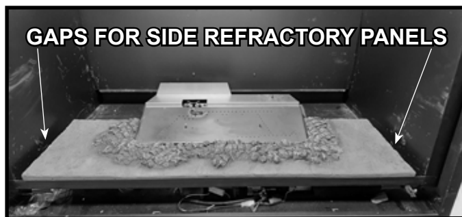
Figure 2 Base Refractory Installed
