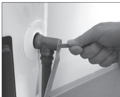
Figure 41 - T&P Relief Valve
