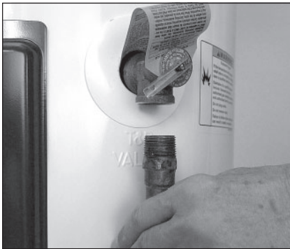
Figure 11 - Removing the T&P Relief Valve discharge pipe.
