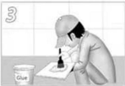
Step 3: Apply glue on the panel back.
