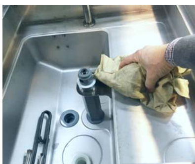
Wipe with a cloth the tank and check for any debris on the bottom.
