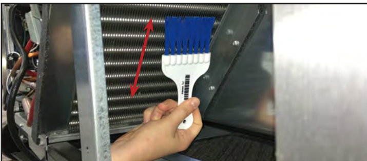
Fig. 3. Never brush across the coil fins.
