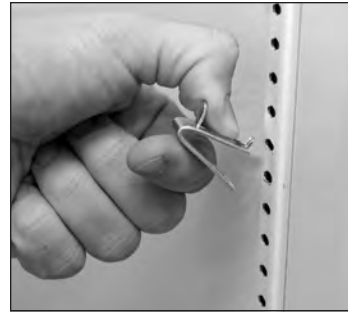
Fig. 1. Installing top tab of shelf clip.
