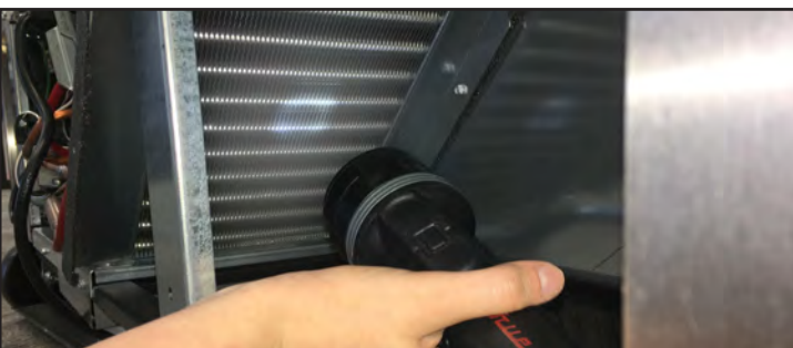
Fig. 4. Verify all blockages have been removed.
