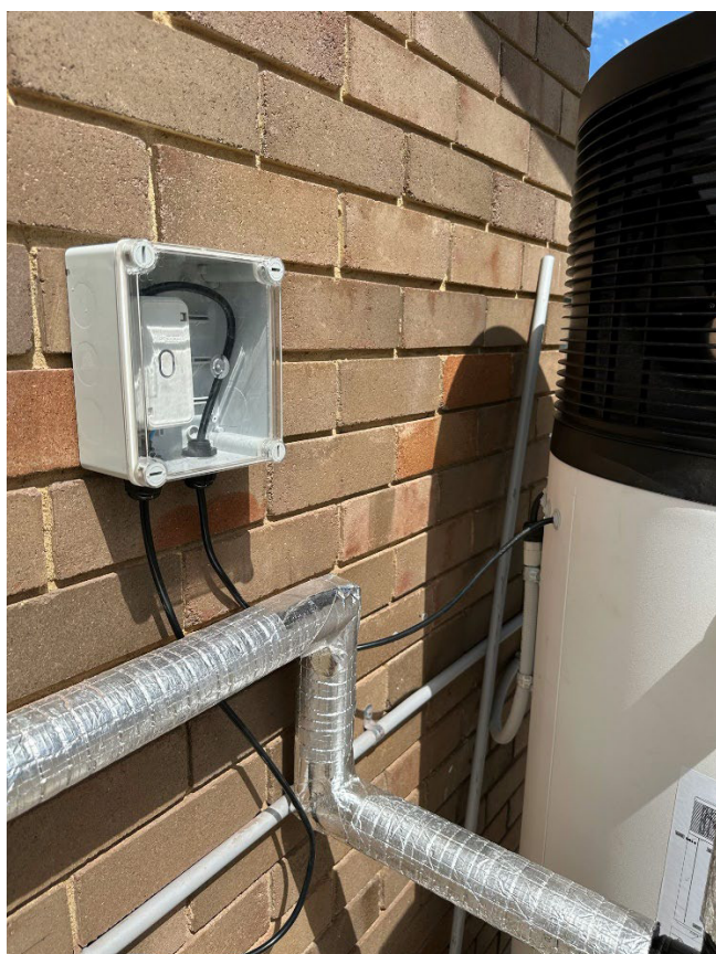
Figure 3. Relay switch signal control
