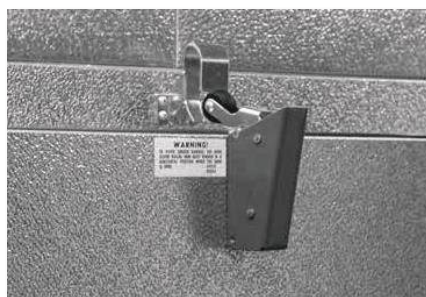
Roller Too High
