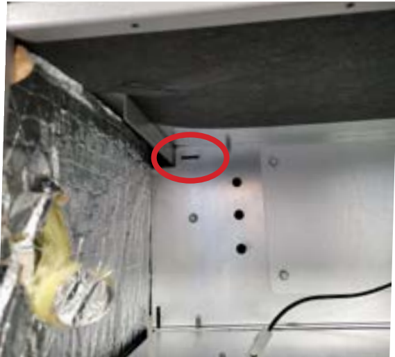
Figure 5. Notch for Control Panel Relocation
