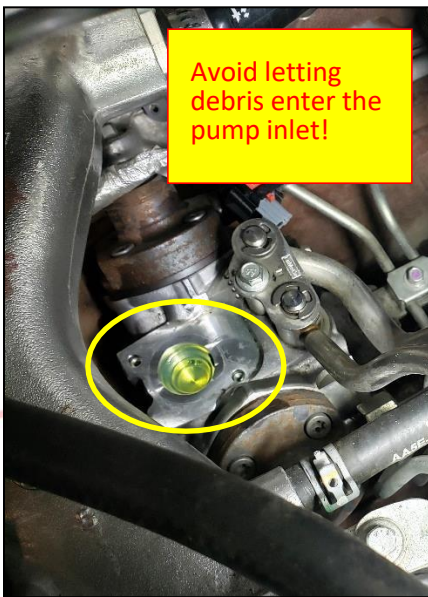
Figure 8: FCA Removed (no debris)
