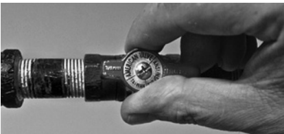
Figure 41: Gas valve in "on" position
