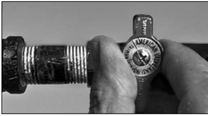
Figure 52: Gas valve in “off” position.
