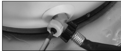
Figure 47: Draining the water heater.
