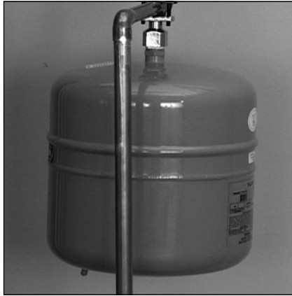
Figure 36: The Thermal Expansion Tank should be pressurized with air, using a hand pump, to match the home's incoming water pressure.
