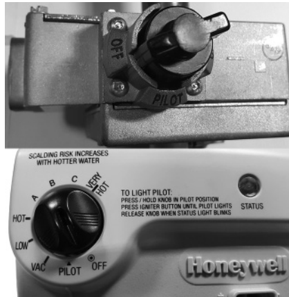
Figure 9: Turn gas control/temperature knob OFF.
