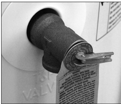
Figure 32: Temperature and Pressure Relief Valve
