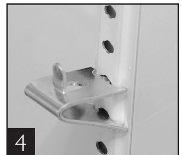
4 Shelf clip installation complete
