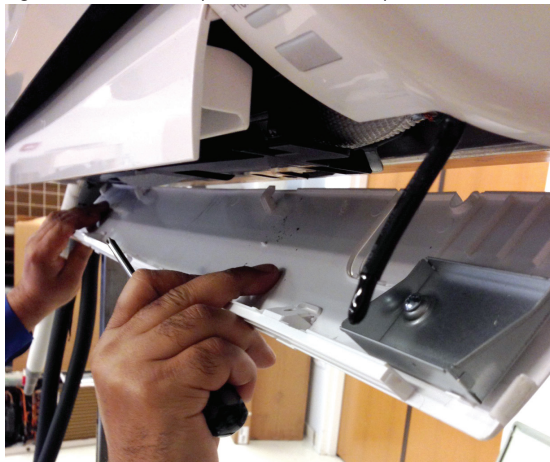
Figure 56: Removal (and Reattachment) of Bottom Panel
