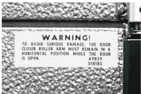
A warning label is affixed to the door section as a reminder.
