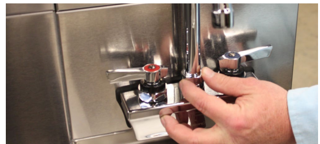
15. Secure the goose neck spout by turning the threaded retention collar clockwise until snug. Finish tightening with an adjustable wrench or channel locks. Do not overtighten.
