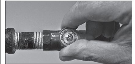
Figure 56: Gas valve in “on” position.
