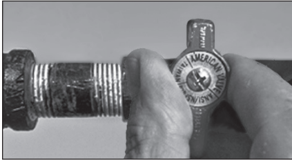
Figure 52: Gas valve in “off” position.
