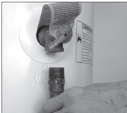
Figure 13: Removing the T&P Relief Valve discharge pipe.
