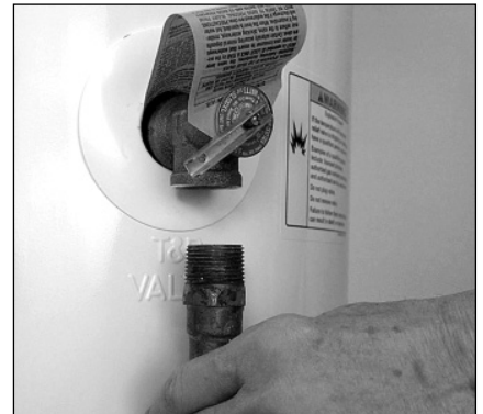
Figure 21 - Removing the T&P Relief Valve discharge pipe.
