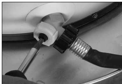
Figure 20 - Draining the old water heater.
