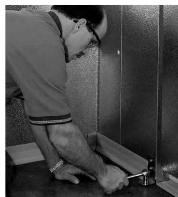
Attach slam brace with fastener provided
