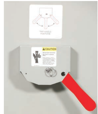
Handle in lockout position
