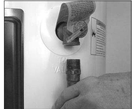
Figure 13 - Removing the T&P Relief Valve discharge pipe.
