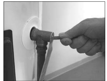
Figure 46 - T&P Relief Valve
