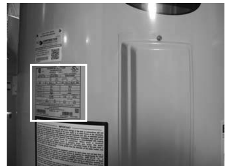
Figure 23 - The water heater’s electrical requirements can be determined from the data plate.
