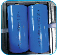
Battery Loading Completed.
