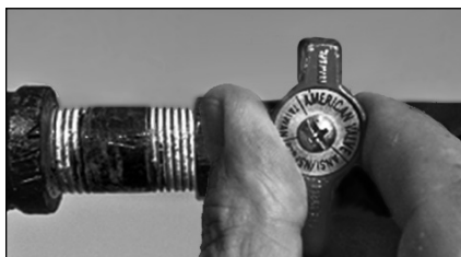
Figure 50 - Gas valve in "off" position.
