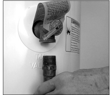
Figure 21 - Removing the T&P Relief Valve discharge pipe.
