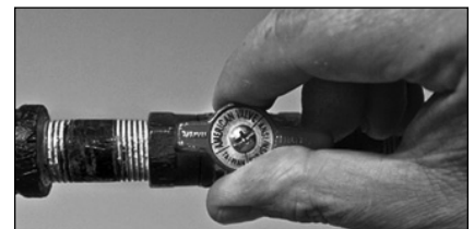
Figure 58 - Gas valve in "on" position.
