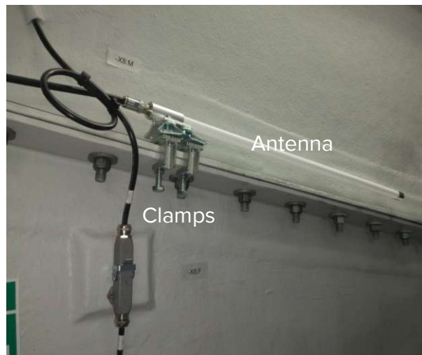
Figure 21 Example of antenna mounting inside with clamps
