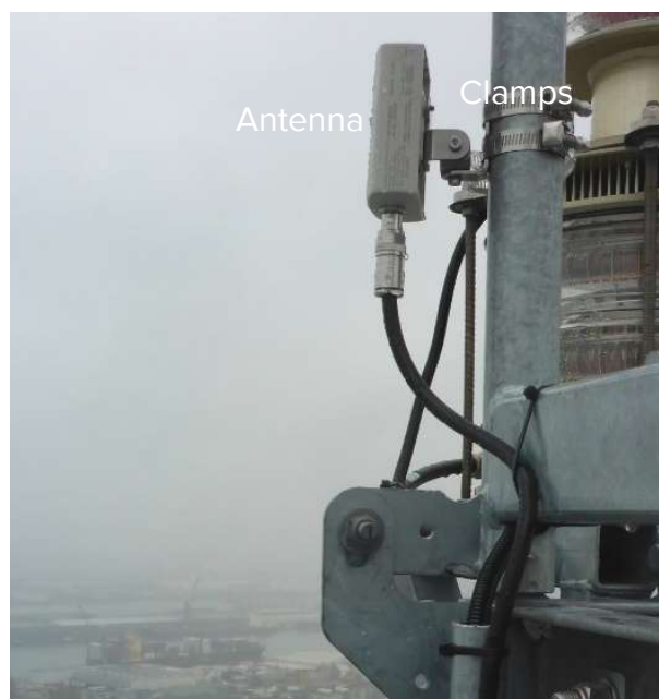
Figure 22 Antenna mounting outside with clamps
