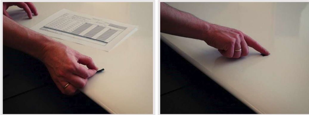
Figure 27 Mark assembly positions
