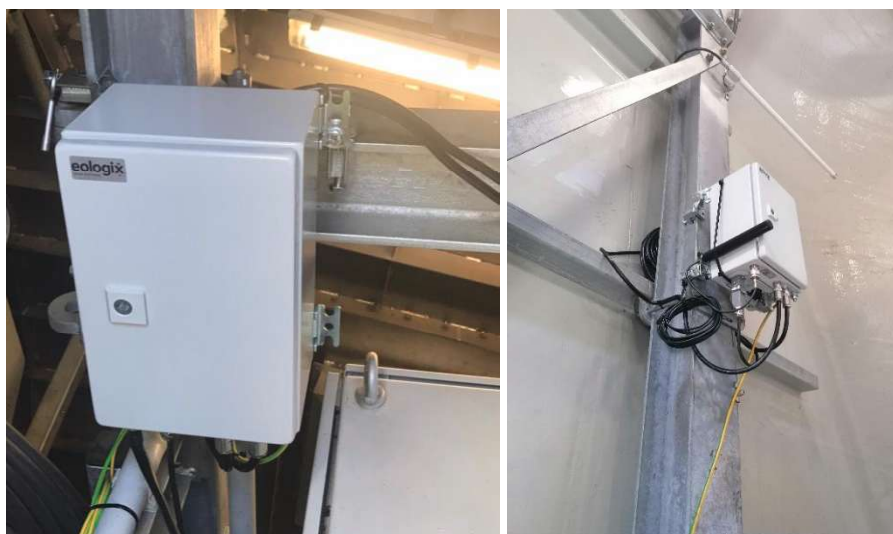
Figure 18 Example of an installed base station (previous version)
