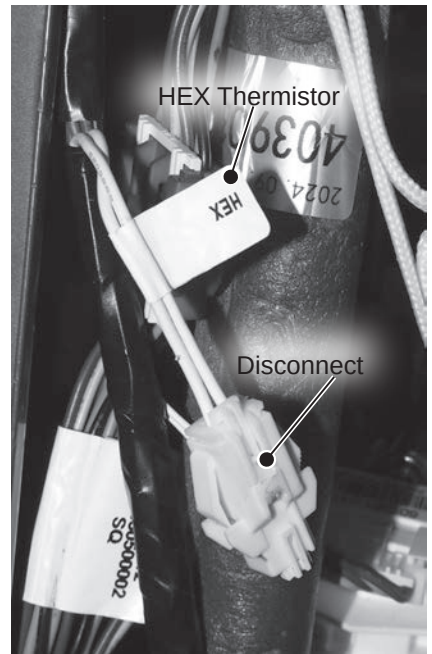
Figure 43 - Disconnecting HEX thermistor
