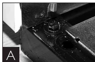
Removing skid from bottom of cabinet.
