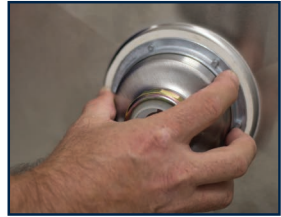
3. Screw on Die Cast Nut and Tighten
