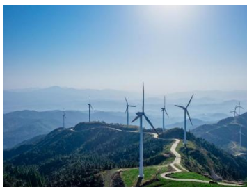
Energy and Power
