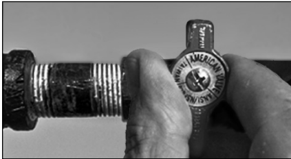
Figure 50 - Gas valve in "off" position.
