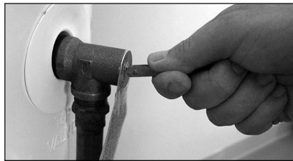
Figure 45 - T&P Relief Valve.
