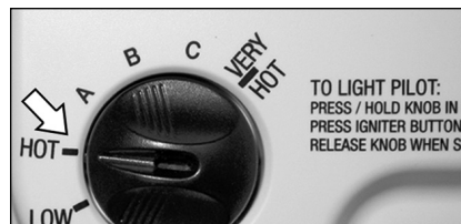
Figure 36 - Adjust the gas control knob to "HOT".
