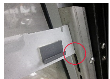
Bottom notch installed (no gap)
