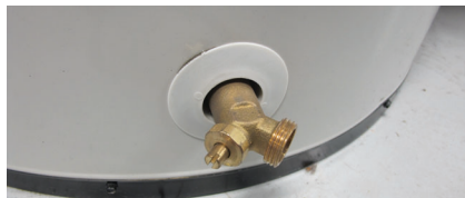
Figure 42 - Drain Valve
