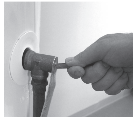
Figure 46 - T&P Relief Valve
