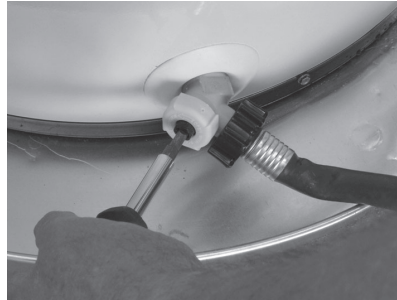
Figure 12 - Draining the old water heater.
