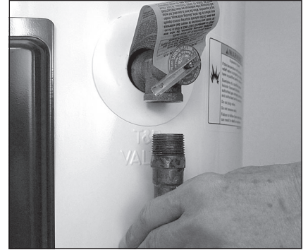
Figure 13 - Removing the T&P Relief Valve discharge pipe.
