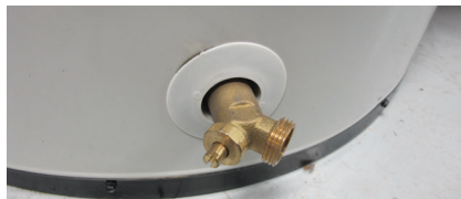
Figure 42 - Drain Valve
