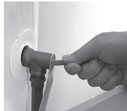
Figure 46 - T&P Relief Valve
