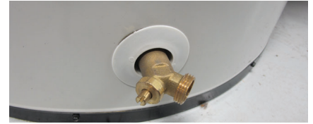
Figure 33 - Drain Valve
