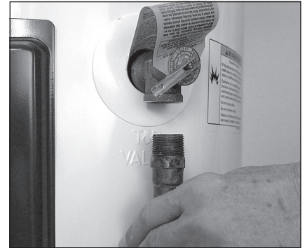
Figure 13 - Removing the T&P Relief Valve discharge pipe.
