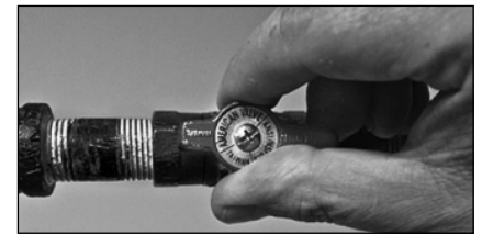
Figure 42 - Gas valve in "on" position.
