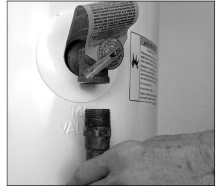
Figure 20 - Removing the T&P Relief Valve discharge pipe.
