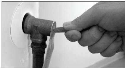
Figure 40: T&P Relief Valve.
