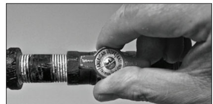
Figure 47: Gas valve in "on" position.
