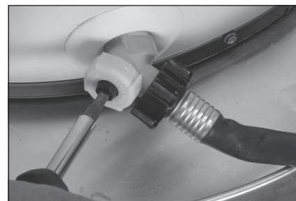
Figure 12: Draining the old water heater.
