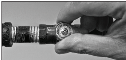
Figure 29: Gas valve in "on" position
