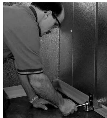
Attach slam brace with fastener provided
