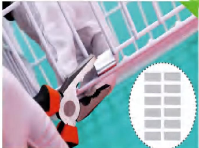
Secure with metal sheets
