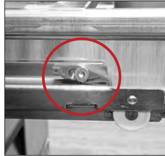
Fig. 5. Drawer retainer location. Retainer is engaged.
