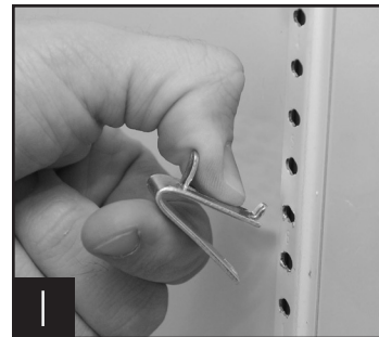
1 Installing top tab of shelf clip
