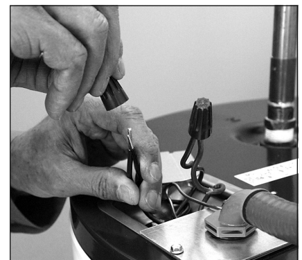
Figure 19 - Connecting the electrical wires.
