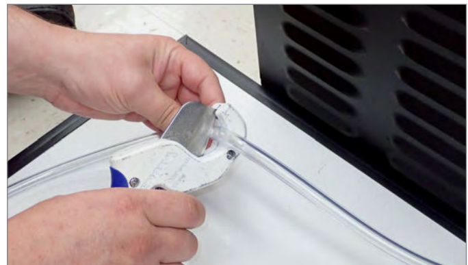
FIG. 3. Cut the drain line with tubing cutters.
