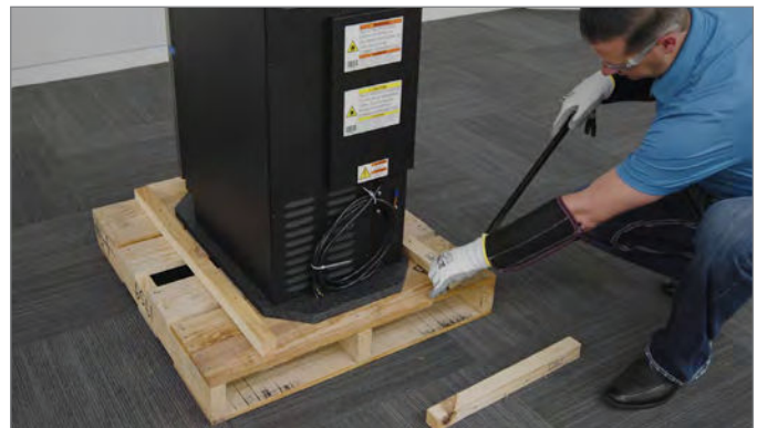
FIG. 2. Pry the runner boards off the skid.
