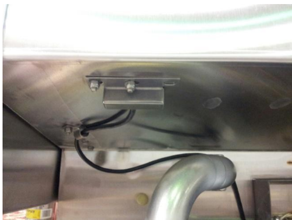
Sequence reed switch for wash tank
